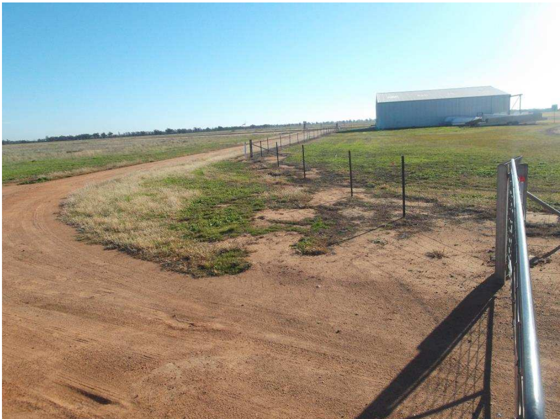
Plate 14: General alignment of the roadway that will provide access to the restricted airside lots.
