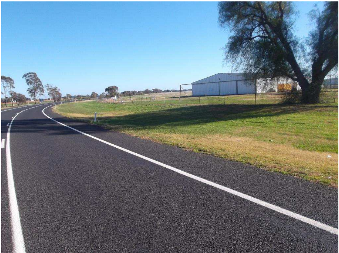
Plate 6: Mitchell Highway looking westbound with an existing aerodrome hangar in the background.
