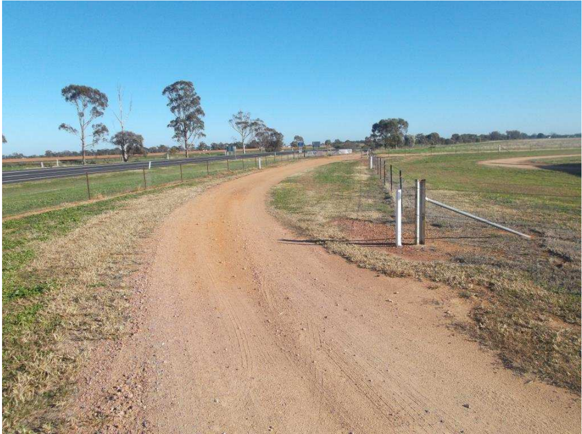
Plate 13: Aerodrome Perimeter Road parallel to the Mitchell Highway.
