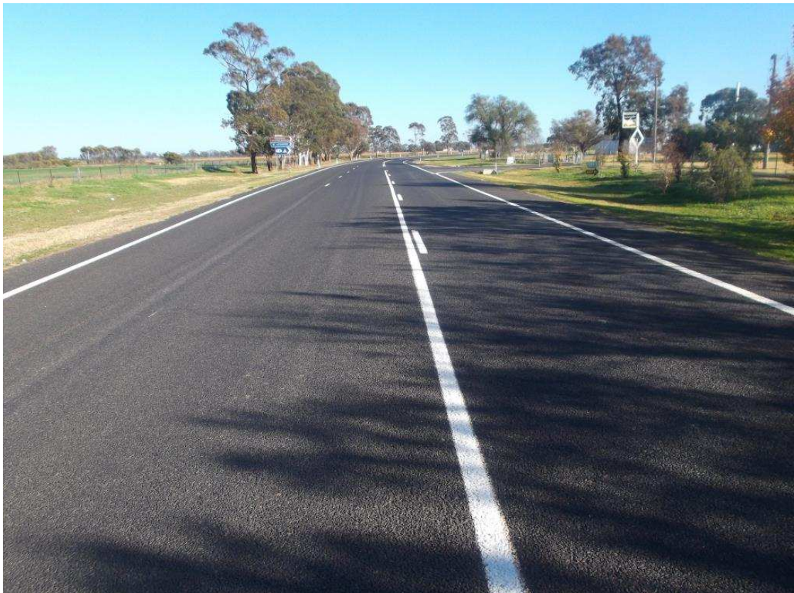
Plate 2: Mitchell Highway looking westbound with the roadway tapering to the full width AUR turning and passing lanes.
