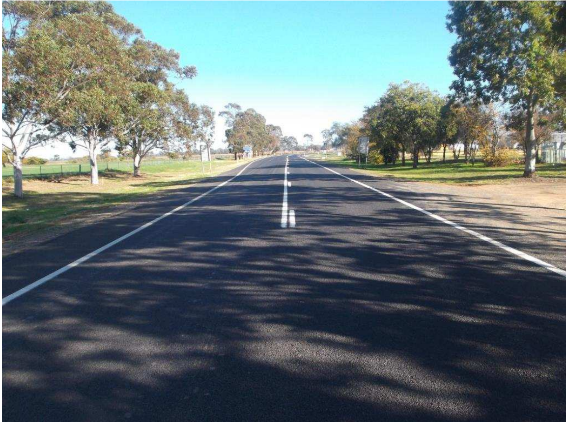
Plate 1: Mitchell Highway looking westbound approaching the intersection access to the Narromine Aerodrome.
