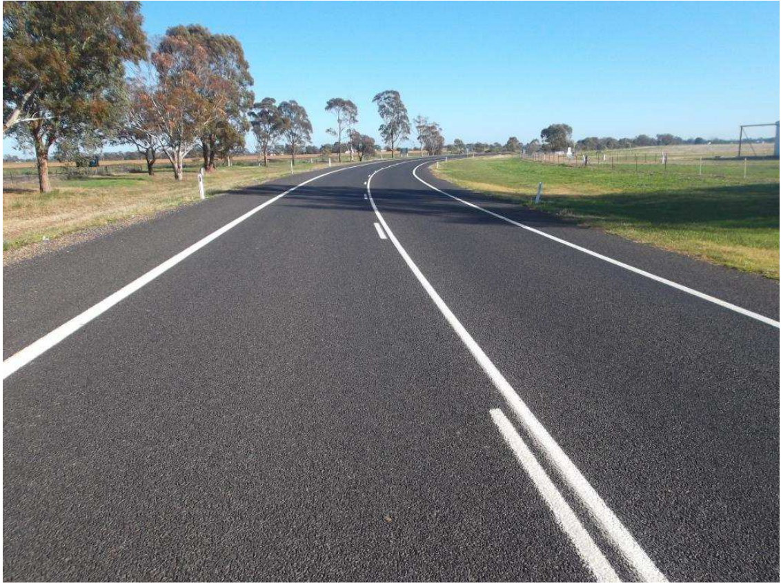
Plate 7: Mitchell Highway looking westbound west of the merging taper on the departure side of the AUR intersection.
