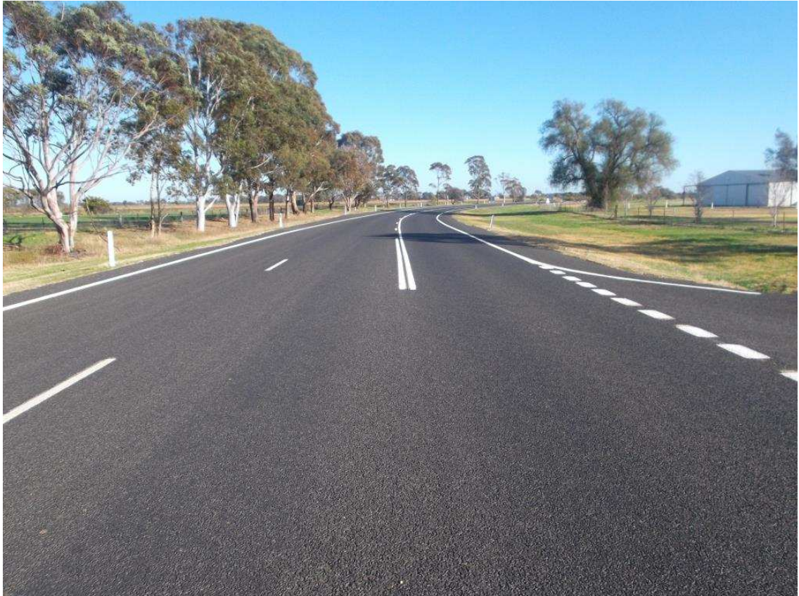
Plate 5: Mitchell Highway looking westbound departing the intersection with Tom Perry Drive.
