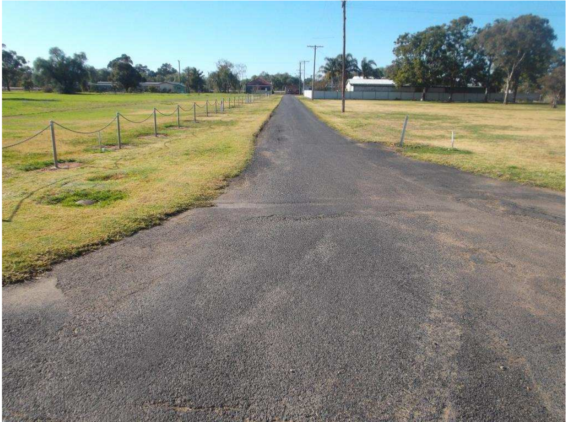
Plate 11: Access road to the Narromine Tourist Park.
