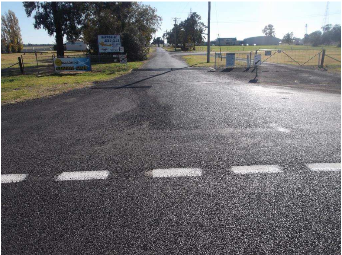
Plate 8: Intersection entrance to Tom Perry Drive showing the existing hold line on the pavement, flaring of the intersection turnout and the cattle grid.
