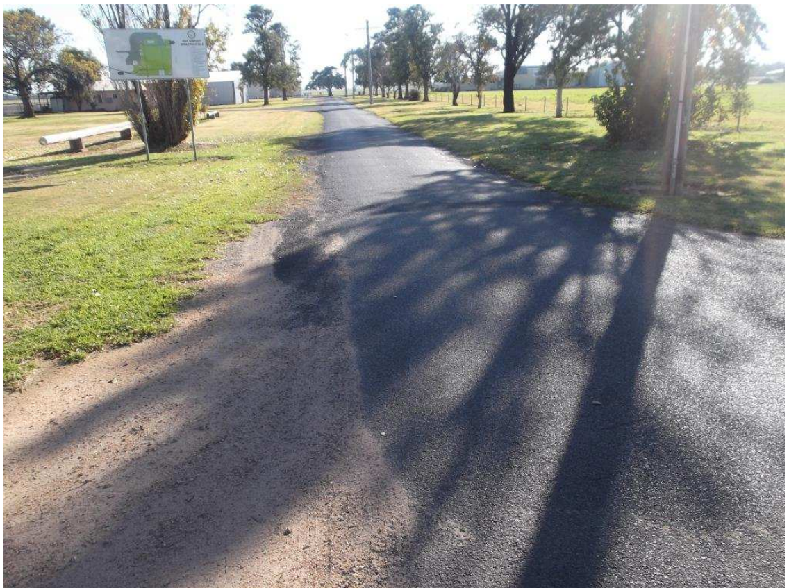
Plate 10: Tom Perry Drive north of the intersection with the Aerodrome Perimeter Road.
